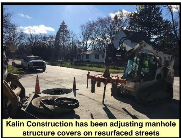
**Kalin Construction has been adjusting manhole structure covers on resurfaced streets**
